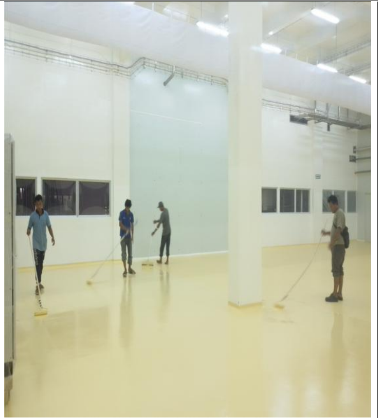
EPOXY FLOORING SIKAFLOOR 263 CREAM (KODE RAL.1001)
