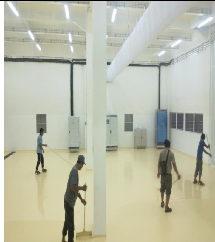
EPOXY FLOORING SIKAFLOOR 263 CREAM (KODE RAL.1001)
