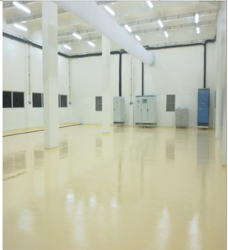
EPOXY FLOORING SIKAFLOOR 263 CREAM (KODE RAL.1001)
