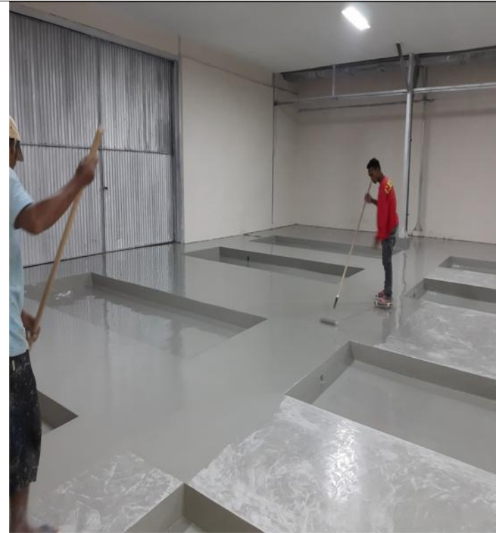
EPOXY FLOORING SIKAFLOOR 263 GREY (KODE RAL.7030)
