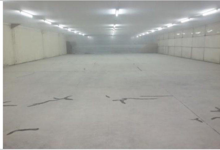
TAHAP-1 : GERINDING & CUTTING CONCRETE EKSTING KEMUDIAN CLEANING AREA SETELAH DI GERINDING & CUTTING
