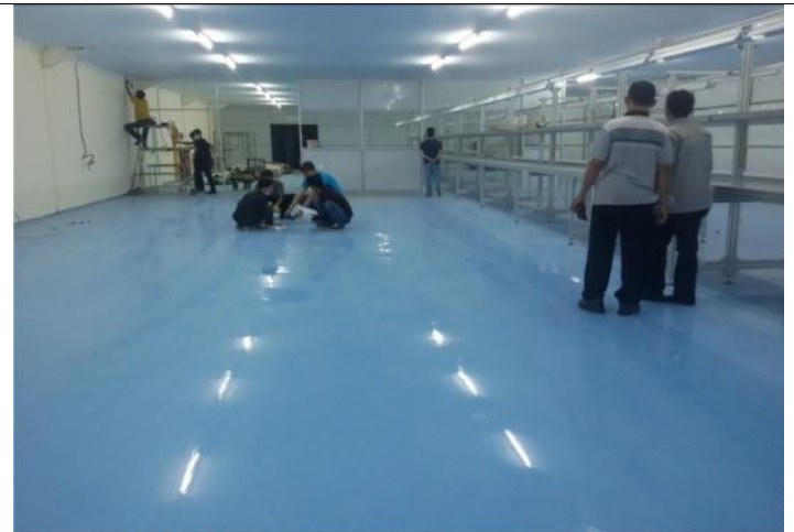
TAHAP-15 : TEST UJI GROUND RESISTANCE (Ohm) & FRICTION VOLTAGE (Volt)
