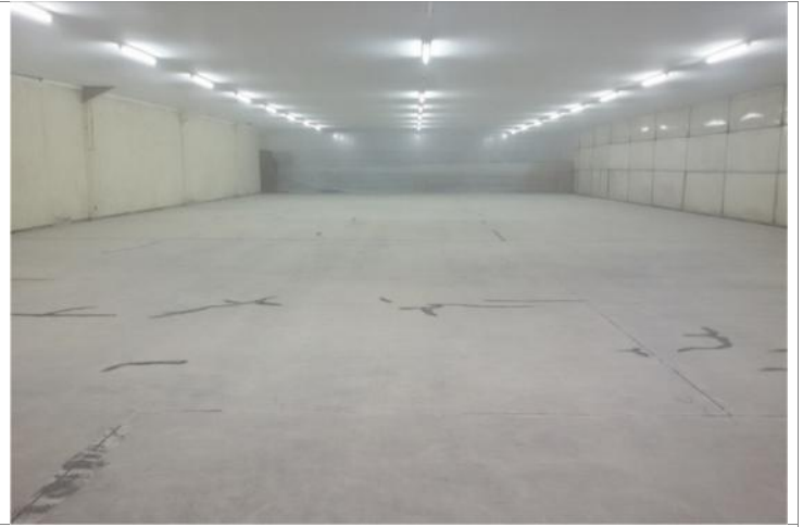
TAHAP-1 : GERINDING & CUTTING CONCRETE EKSTING KEMUDIAN CLEANING AREA SETELAH DI GERINDING & CUTTING
